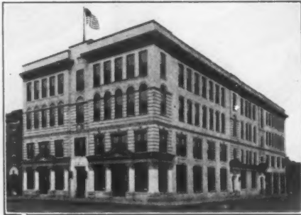
Home Office Building Third and Clay Sts., Richmond, Va.
